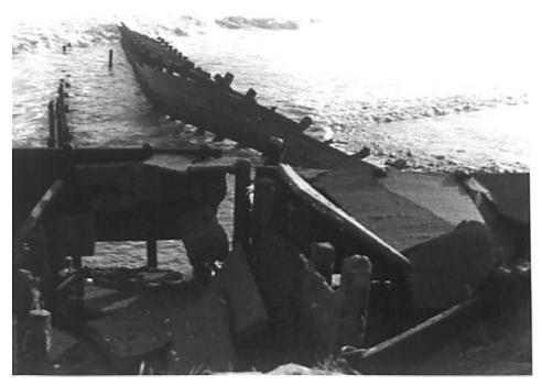
Figure 20 January 1960: collapsed revetment along the Neck – it appears to be fronted by a timber framework and topped with thin concrete slabs (from Phillips 1962)
