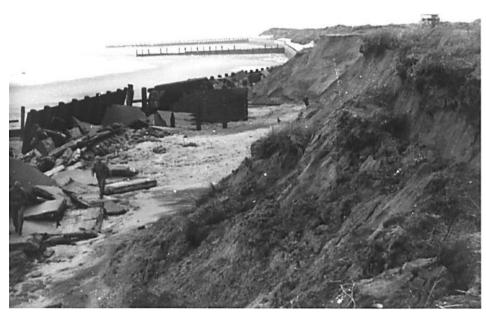
Figure 19 January 1960: Dune erosion behind collapsed revetment along the Neck (from Phillips 1962)
