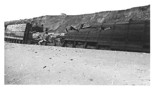
Figure 18 January 1960: Collapsed revetment along the Neck (from Phillips 1962)
